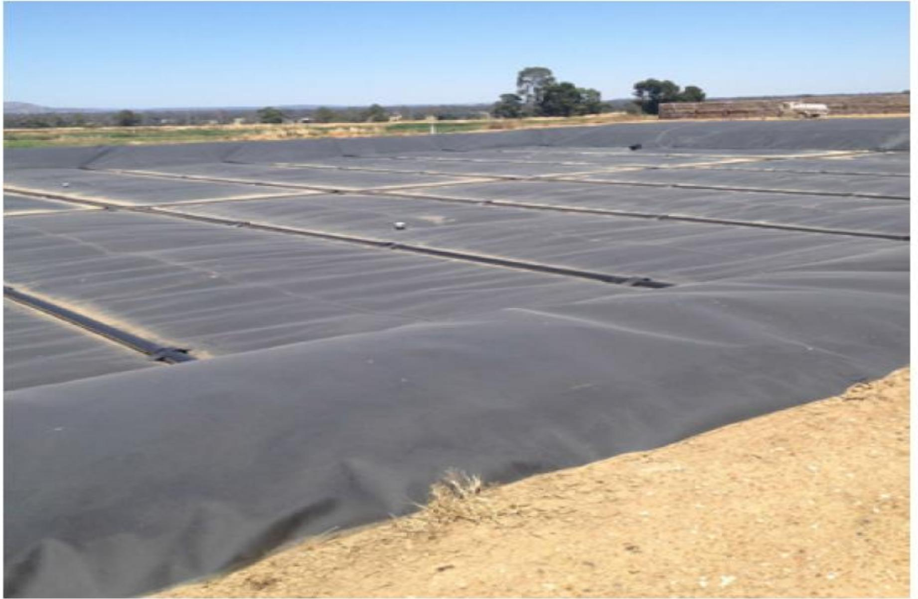
**Covered Anaerobic Lagoon**
