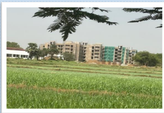
New hostel under construction
