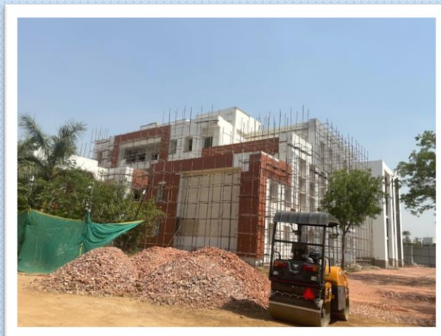
New academic building under construction in the Campus of SGIDT, Patna.
