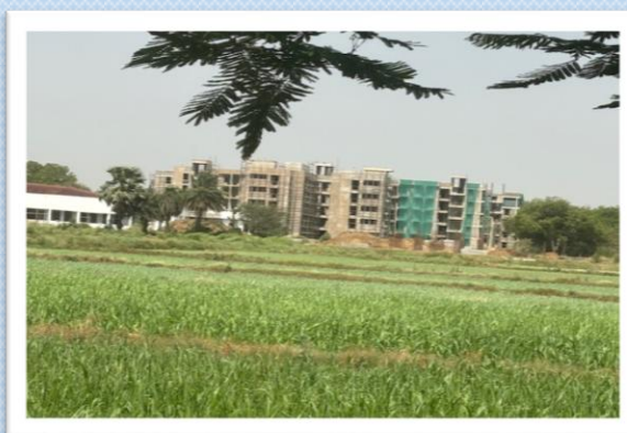
New hostel under construction
